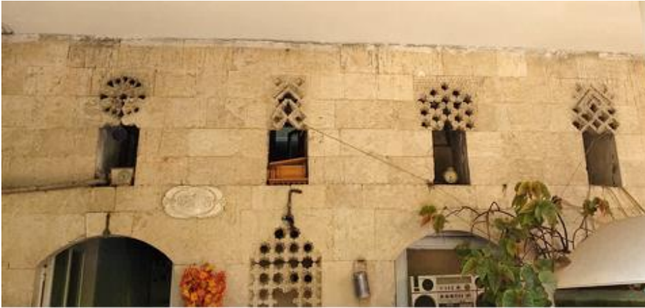
Figure 3.8. Top windows ( kuş takası ) of the studied Ülkü-21 House (Author, 2022)
