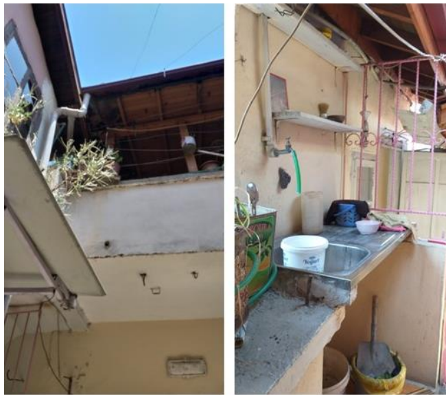
Figure 3.89. The balcony area and the kitchen sink addition (Author, 2022)
