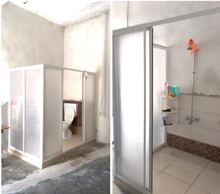
Figure 3.21. The wet space addition with a toilet inside a shower area (Author, 2022).
