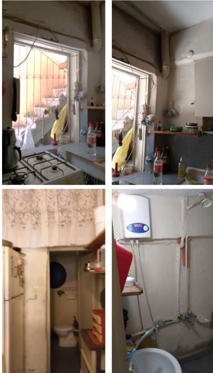
Figure 3.85. The service spaces in 40 Asırlık-65 House (Author, 2022)
