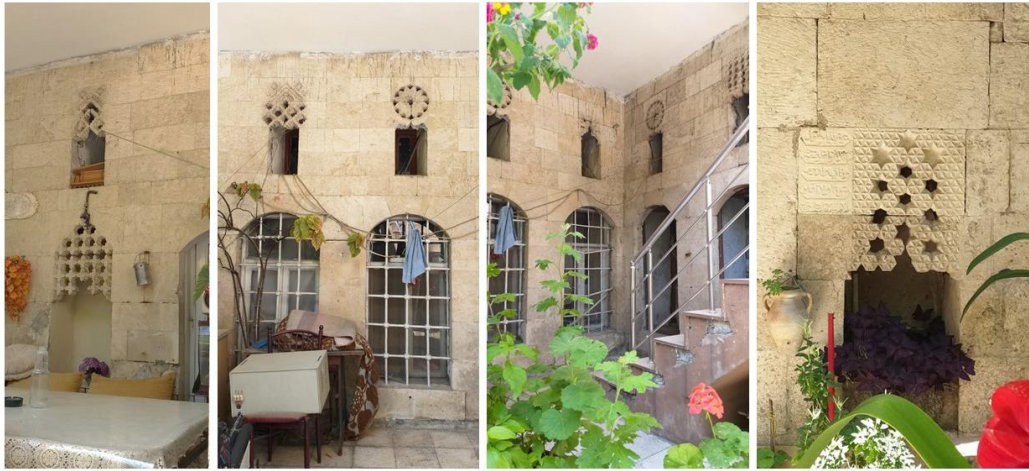
Figure 3.37. Traditional top windows and niches on the front façade of the Ülkü-17 House (Author, 2022)
