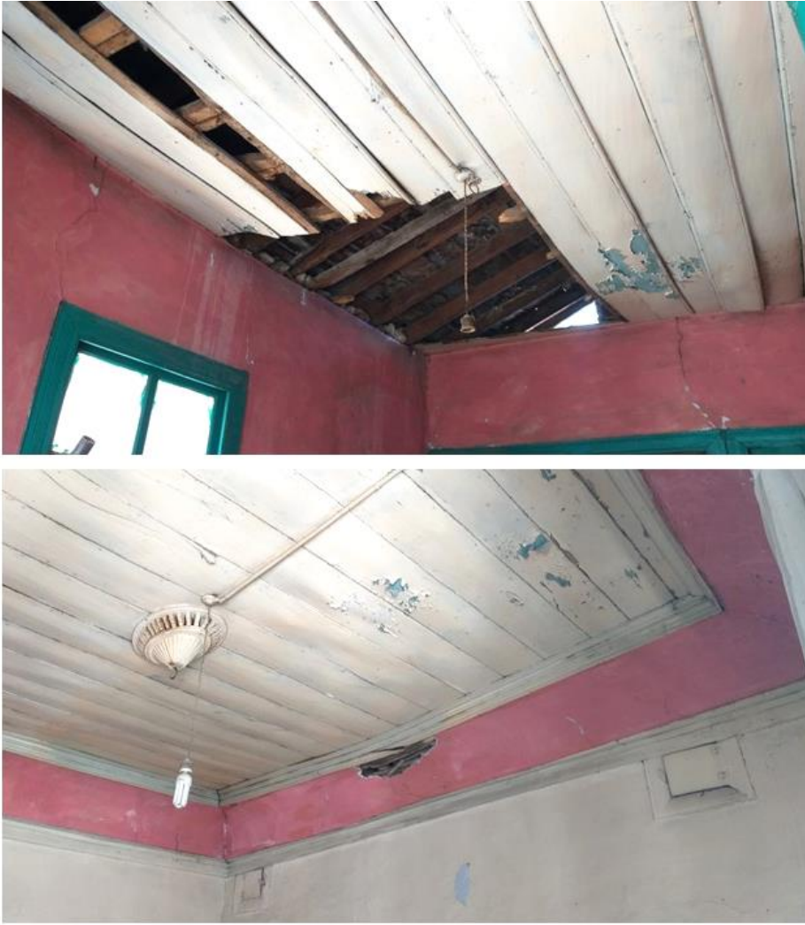
Figure 3.30. The ceilings of the first-floor rooms of the Mass B (Author, 2022)
