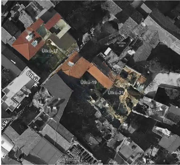
Figure 5.2. Part of Ülkü Street after the Earthquake (Retrieved from atlas.hgm.org.tr)
