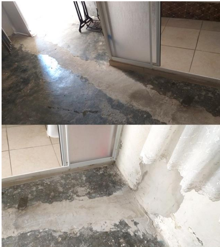
Figure 3.22. Screed covered traces on the concrete slab of the room (Author, 2022)
