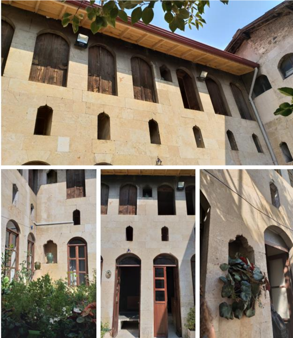
Figure 3.67. Traditional façade elements of Asi House (Author, 2022)
