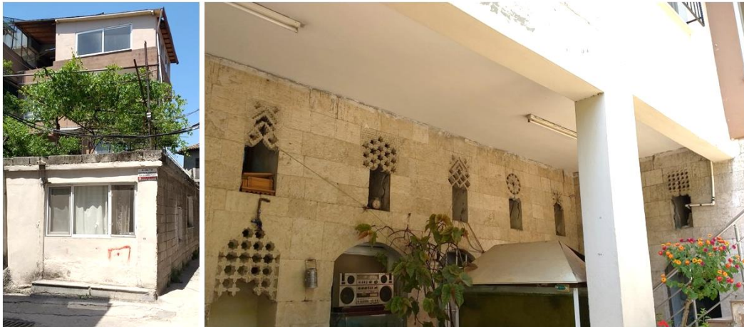
Figure 3.39. The upper floors of Ülkü-17 House constructed with new techniques (Author, 2022)
