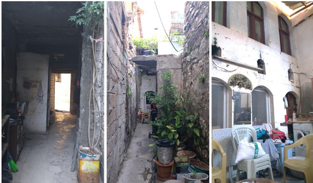
Figure 3.40. The lot, the entrance and the façade of Ülkü-5 House (Author, 2022)
