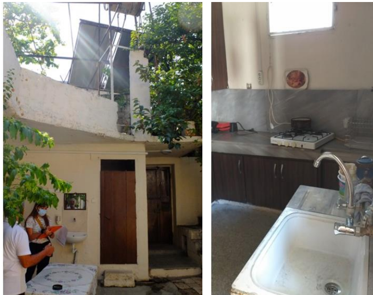
Figure 3.72. The WC addition, the flat roof with the solar panels, and the kitchen in Asi House (Author, 2022)
